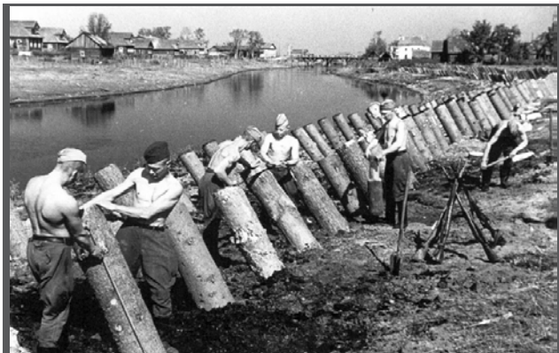
August 20, 1942. The troops of the Volkhovsk Front are building the anti-tank barricade
